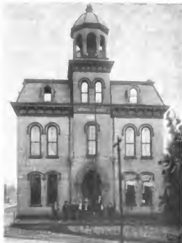
CITY HALL, EAST LIVERPOOL
